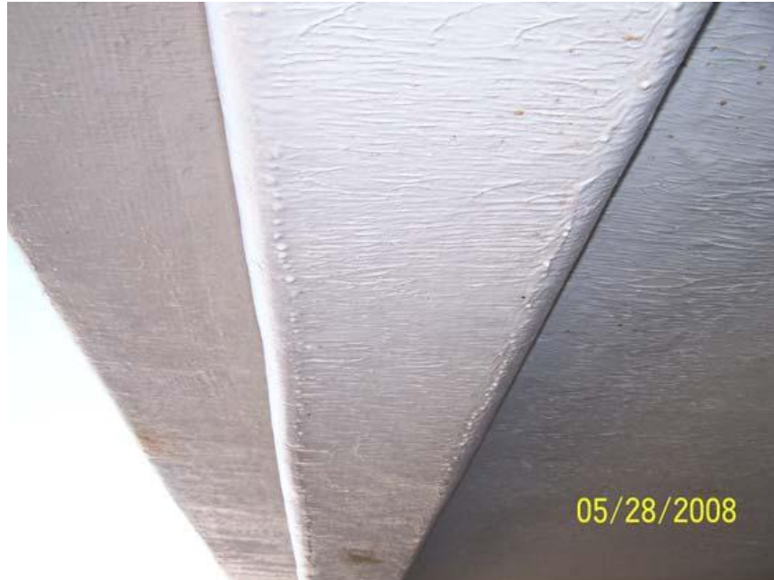
Figure 8: Water droplets formed on the beam. Picture was taken at 10 am., May 28, 2008.
