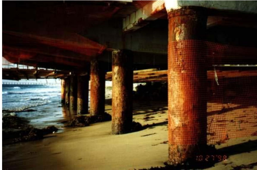
Figure 2: Corroded slab (a), beam (b) and pilings (c).
