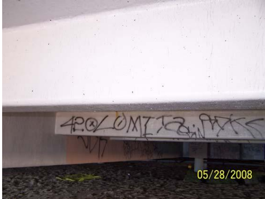
Figure 6: No signs of defect on the beam.
