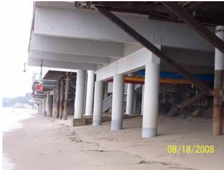
Figure 5: The retrofitted columns and beams on August 18, 2008.
