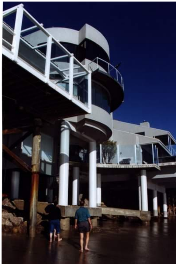
Figure 4: Columns retrofitted with Tyfo® Fibrwrap® System.
