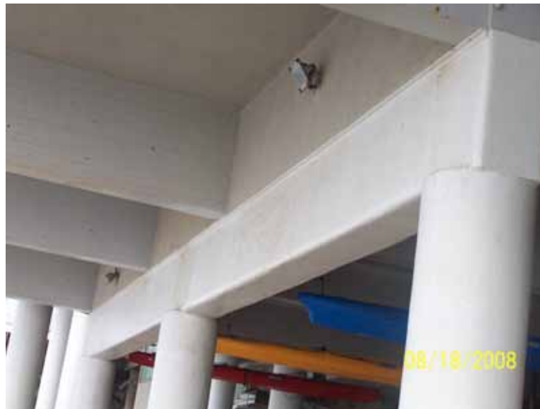
Figure 8: joints between the retrofitted column and the beam
