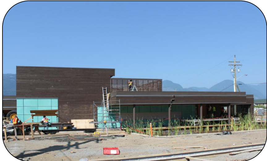
New museum building retrofitted with the Tyfo® Fibrwrap® System
